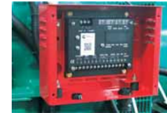
Speed Governor Installed externally for easy future upgrades
