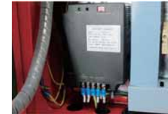
Battery Charger Enables the battery to be in constant recharging in which the generator set can be started at all time
