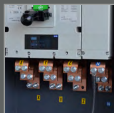
Connection copper bars where provided they allow to connect more cables on the same phase
